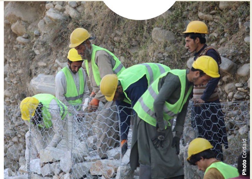
Construction of a protection wall for an irrigation channel implemented through a cash for work project where the local community members are also recruited to work in the project and receive daily wages.
